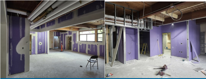
Kitchen: Sheetrocked & Taped
